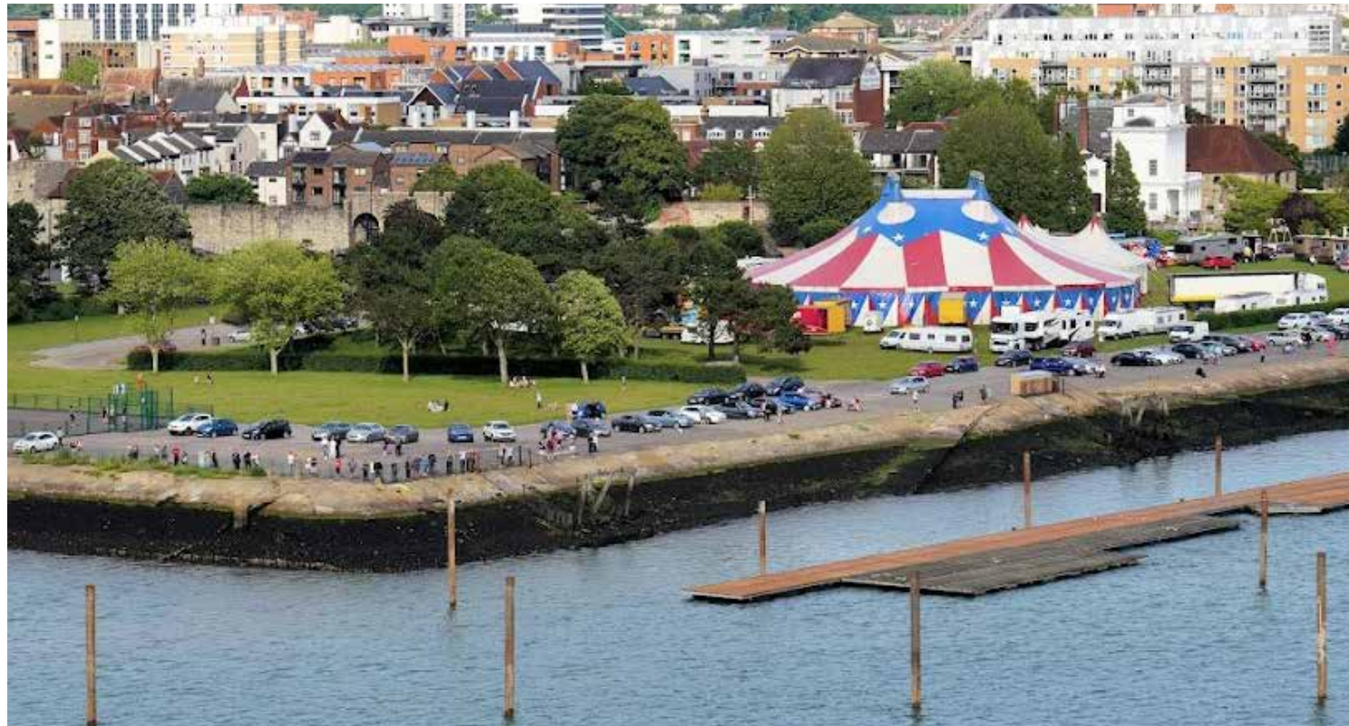
Mayflower Park - Existing waterfront public concourse and revetments to be replaced
