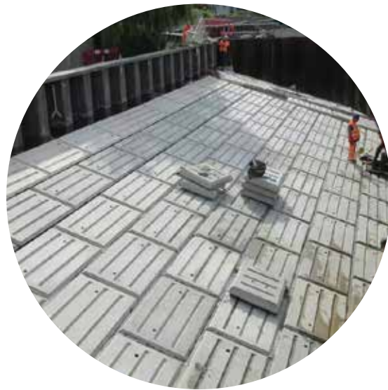
1. Precast concrete revetment canewdon blocks
